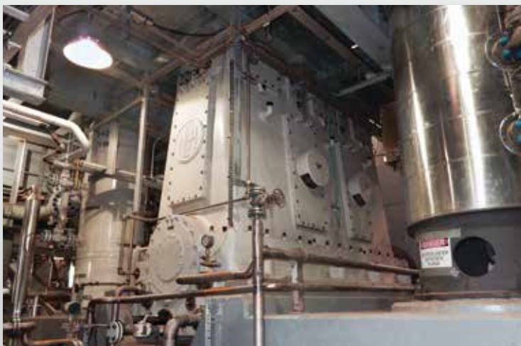
NEA compressor model: 2SVS320 - two stage, lubricated, 4-throw, vertical Application: Gas Processing
