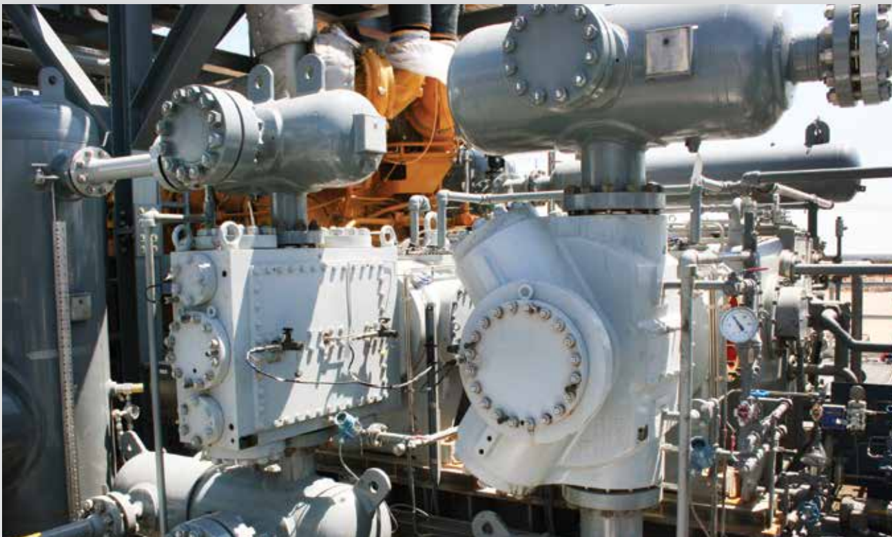
NEA compressor model: 3SVL320hs - three stage, lubricated, 4-throw, horizontal Application: CO 2 Injection for EOR
